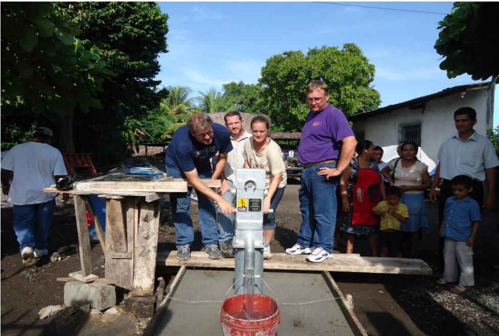
Completed water project accessible by the entire community and will be used to meet their most immediate water needs.
