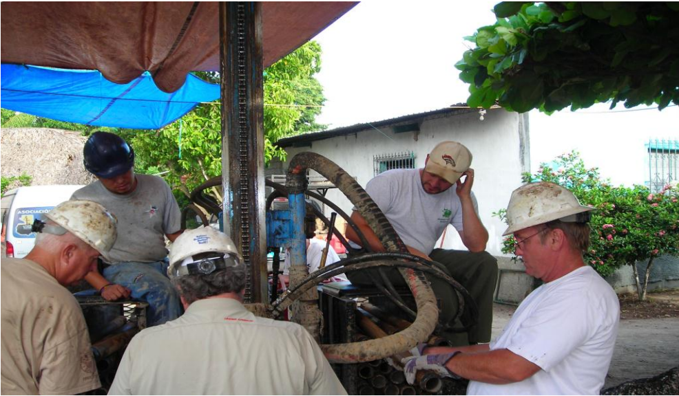
Project in process.
